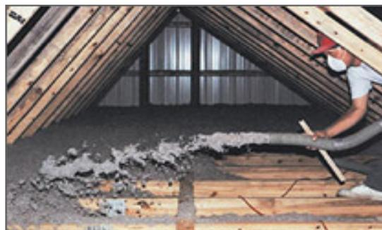
If the existing insulation value is R-11 or lower, it must be brought up to R-30 value).
